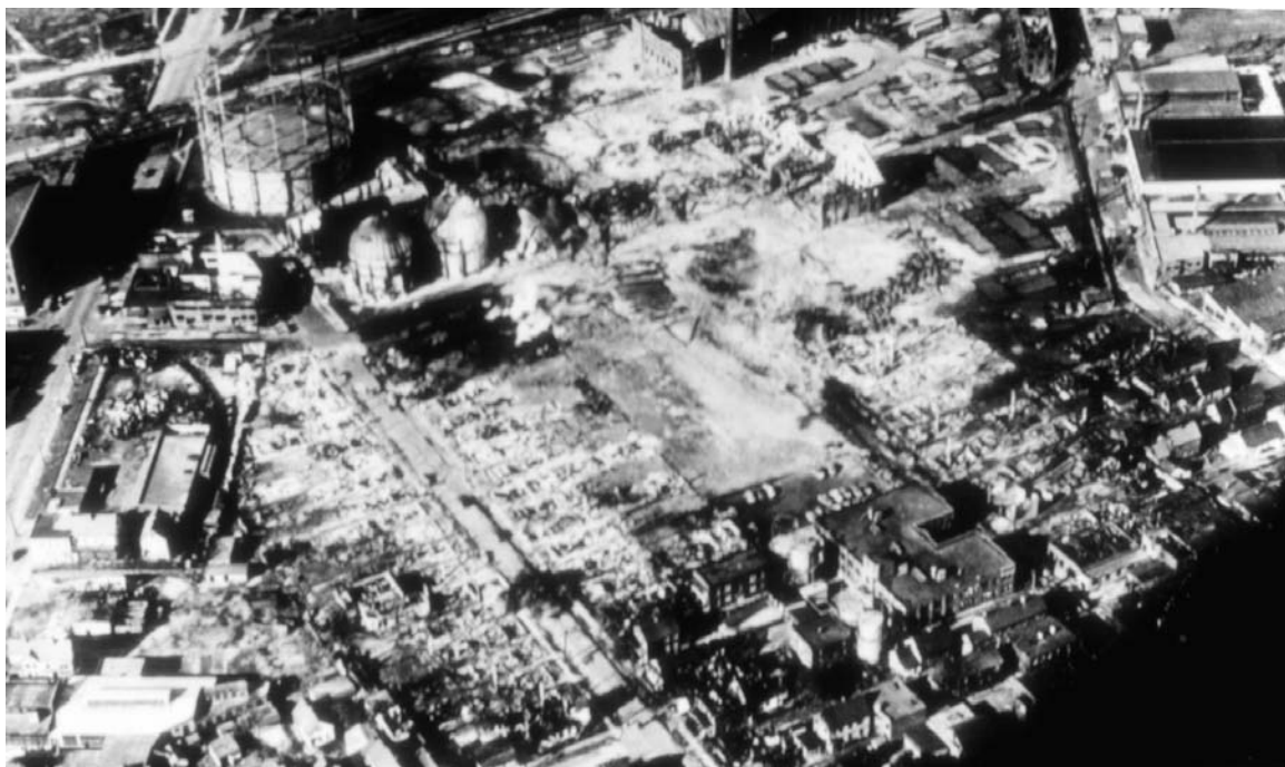
Fig. 9.2 Devastation caused by brittle fracture of liquid natural gas tank in Cleveland, Ohio, Oct 1944
